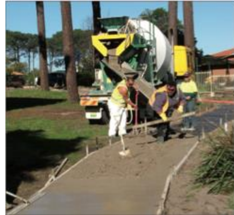
Fly ash geopolymer footpath
