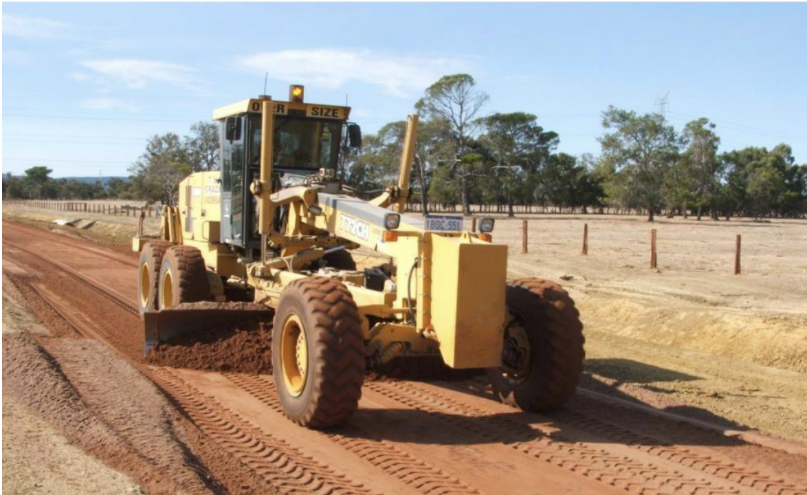
Road construction by Main Roads Western Australia using Red Sand™
